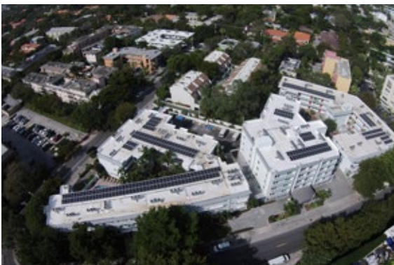
Pictured: Our Residence Inn Coconut Grove Hotel is topped with a 336-panel, 92 kW Solar PV system. The system captures renewable energy from the sun, and generates 150,000 kWh of electricity each year for the hotel. This system provides 10% of the total hotel electricity usage.
